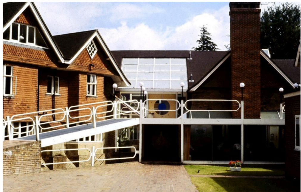
Figure 4. Cullinan Studio, Main Entrance to the extension of Olivetti Training School Haslemere, England, UK. Courtesy and credits of ©Cullinan Studio.
